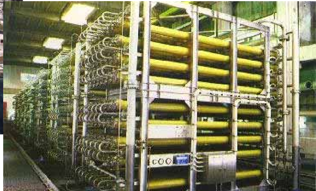
RO Module Installation (each unit produces 5,000m 3 /d)
