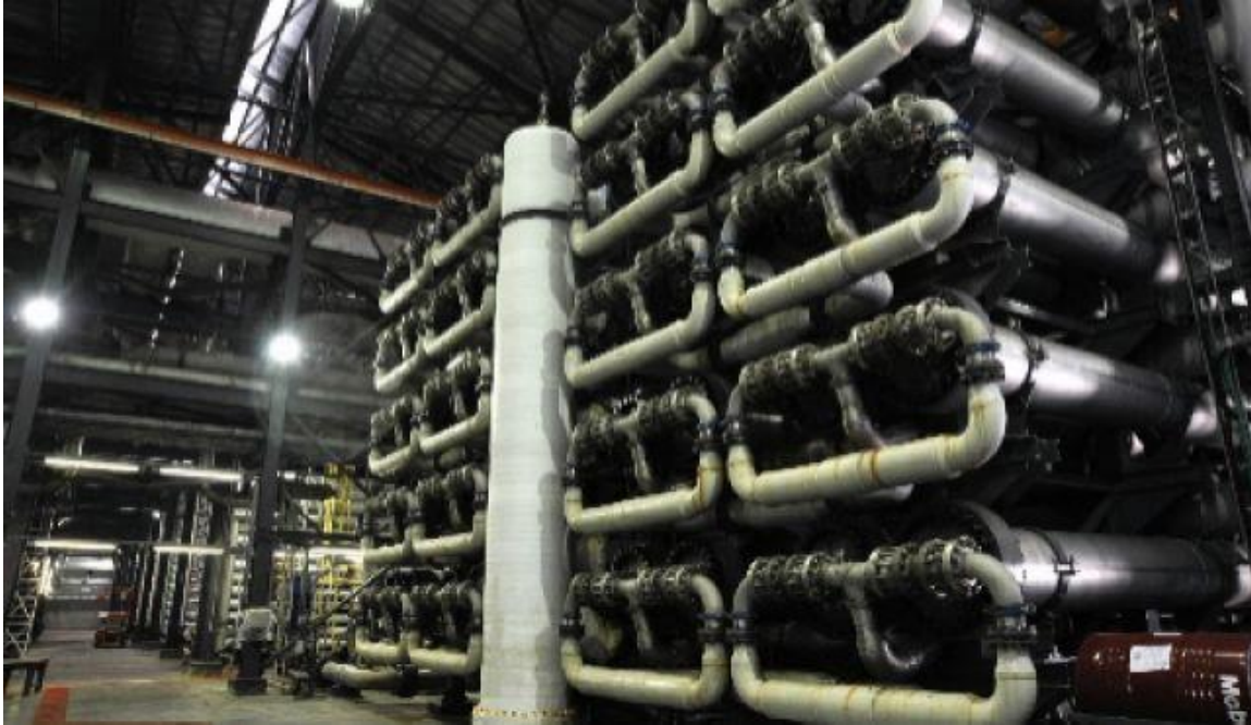
Fig 2.10: DWEER™ system of the Ashkelon seawater plant (Goichon, 2007)
