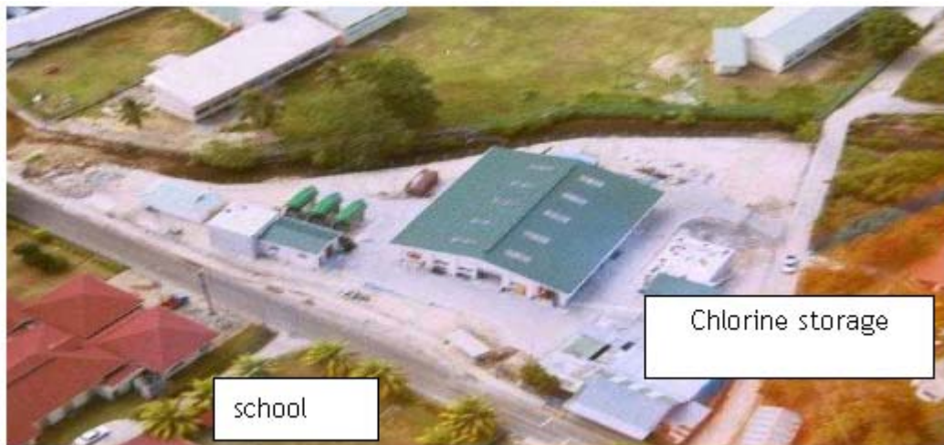
Figure 5. West Coast site.
