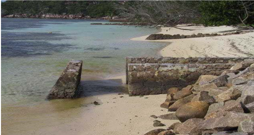
Figure 4. La Digue brine discharge.
