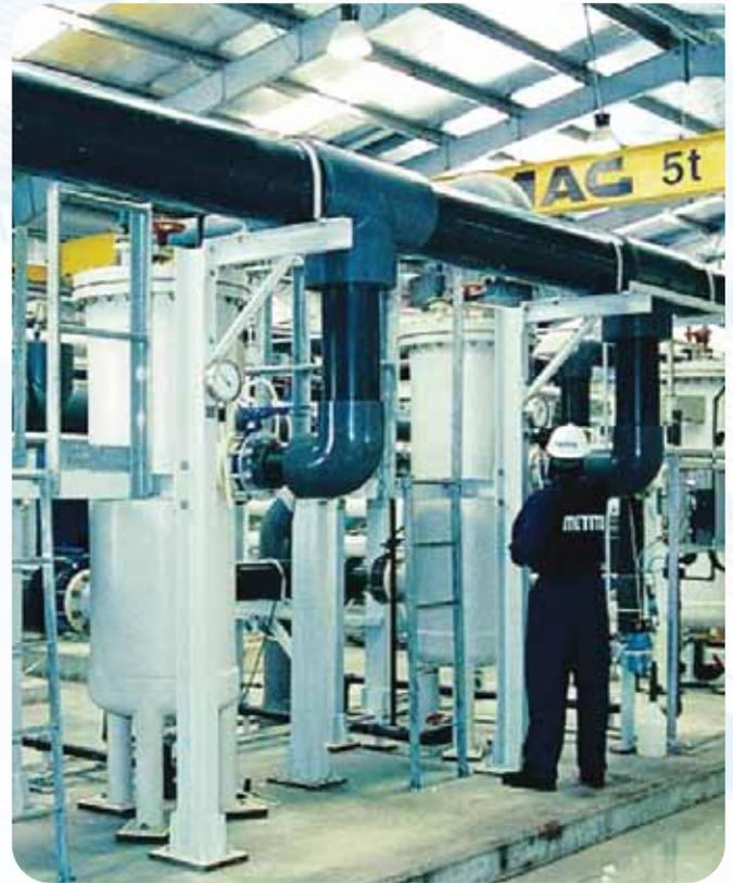
Filtered water from the multi-media filters is further dosed with antiscalant and a dechlorination agent before it is passed through a set of 5-micron cartridge filters followed by another bank with 1-micron particle cut-off rate. Such extensive filtration ensures that feed water to the reverse osmosis membranes has a SDI < 3.
